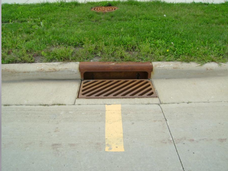
Storm Inlet with Standard Curb & Gutter
