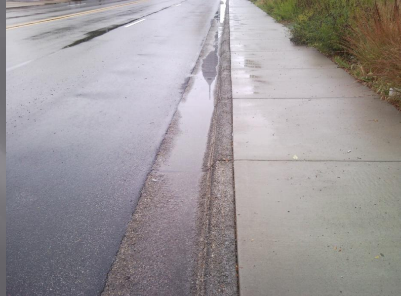
Pervious Curb & Gutter
