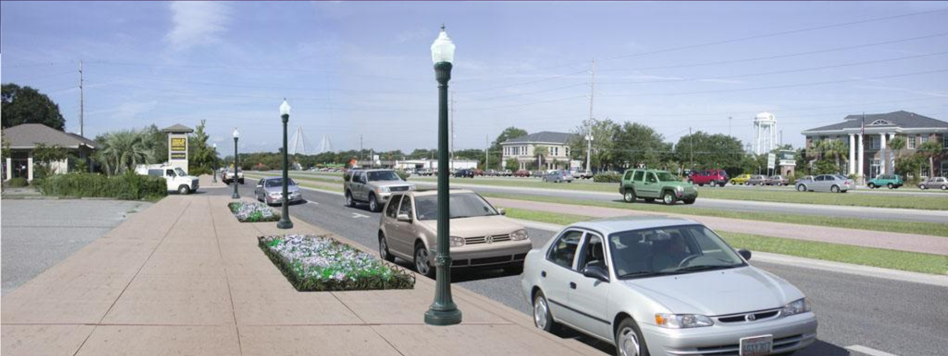
New sidewalks, one-way local access lane, parking lane, street lamps
