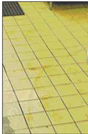
Broken and wet floor tiles.
