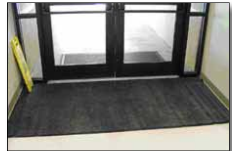
Entrance way with wet carpet.
