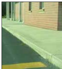
Watch for uneven surfaces and elevation changes between sidewalks and parking lots (roadways).
