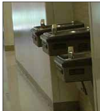
Water fountain area.
