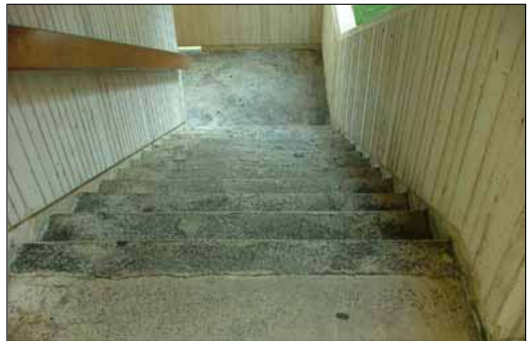
Watch for hazardous conditions on stairs, such as excessive mold and deterioration of the cement.
